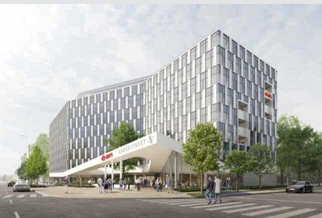
Baker Street Phase 1
